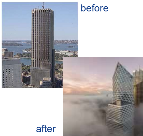
Quay Quarter Tower, Sydney (Australia)
